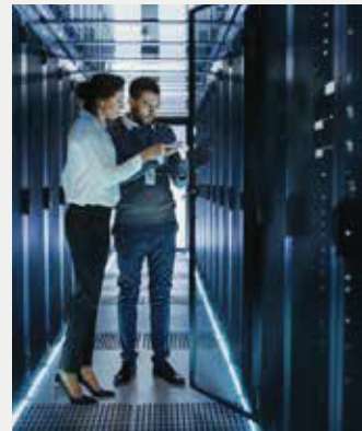
Instant data center
